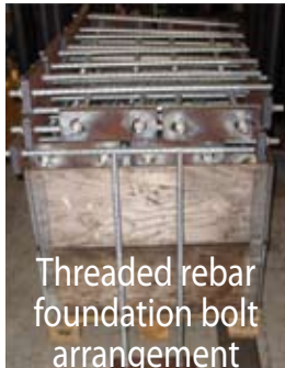
Assembled Holding Down Bolts
